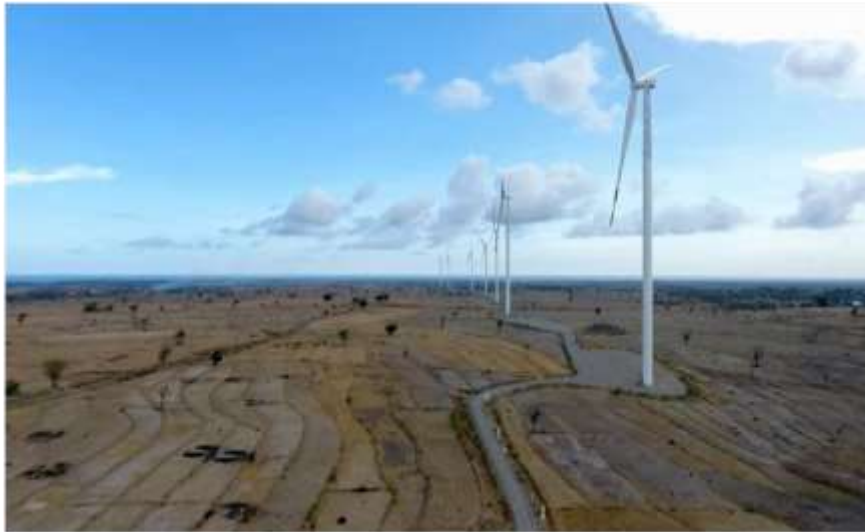
Figure 3: Siemens Wind Turbine Generator
